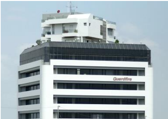
Guardfire Head Office (Guardfire Limited)
